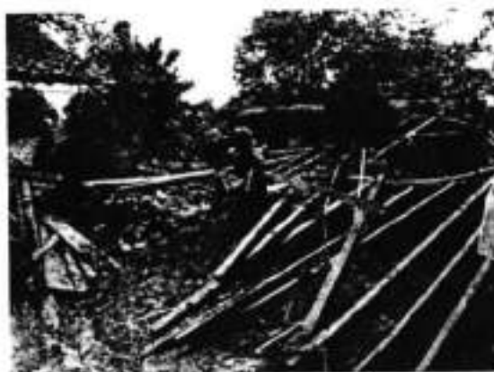
[Fully Damaged house of a Tribal]
